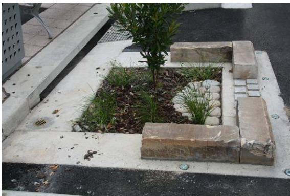
South Street, Granville WSUD elements (clockwise from top left) – centre media bioretention, inlet to median bioretention, street-tree pit, and street-tree pit showing overflow.
