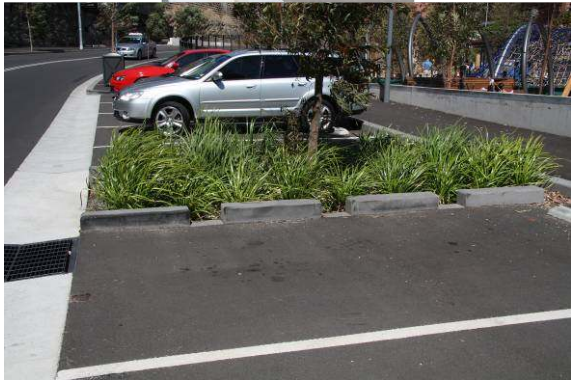
WSUD Elements (Clockwise from top left) – Street tree in Pirrama Road, central spine bioretention system, bioretention system at base of cliff on southern end of park, carpark bioretention systems.
