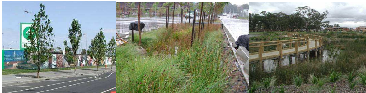
Figure 1.: Street trees that collect and treat runoff from Bourke St, Melbourne (left), the rain-garden in Victoria Park, Sydney (middle) and Lynbrook Estate stormwater wetland, Melbourne (right).
